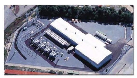
Typical compact (voltage sourced) HVDC converter station and (outdoor substation)
