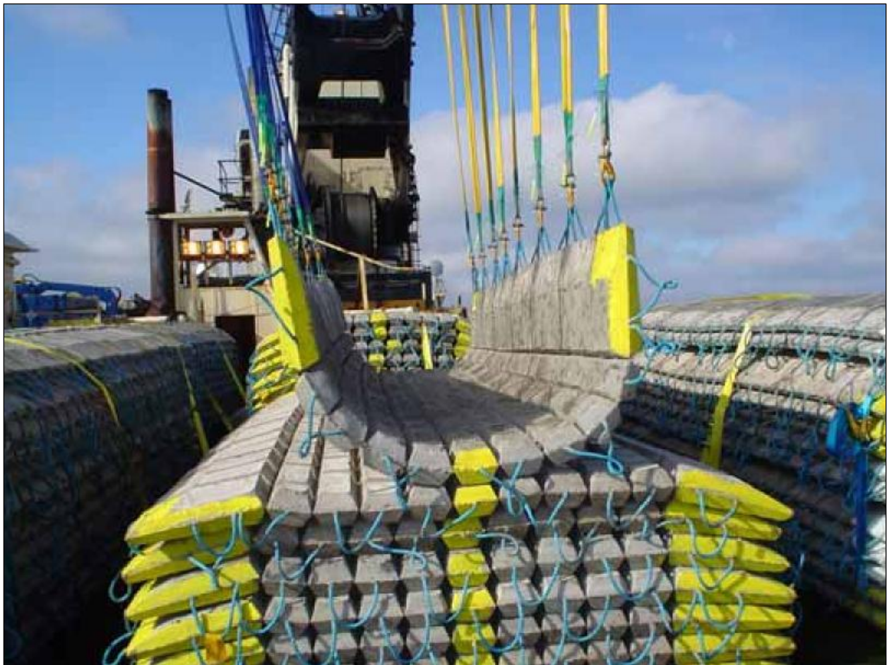
Figure 2-7. Typical Articulated Concrete Mats
